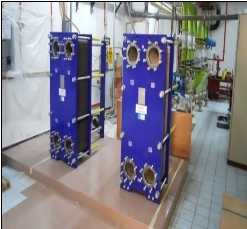
Fig. 11. Installation of plate heat exchanger
