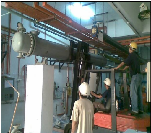
Fig. 6. Dismantling of Shell and Tubes Heat Exchanger
