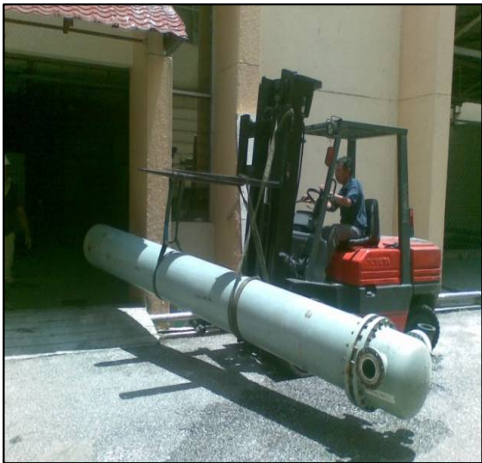
Fig. 7. Removing the Heat Exchanger from Basement
