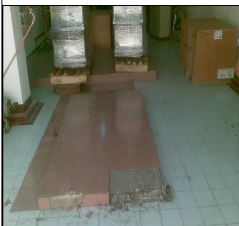
Fig. 10. Construction of new concrete plinth concrete Support
