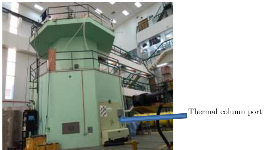
Figure 1: Reactor at RTP showing thermal column location.
